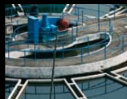
Waste Water Treatment Plants
